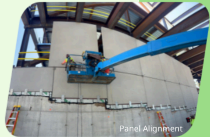
Panel Erection
